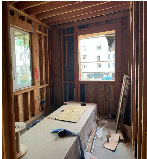
Area S5 - View of unit November 12, 2025
