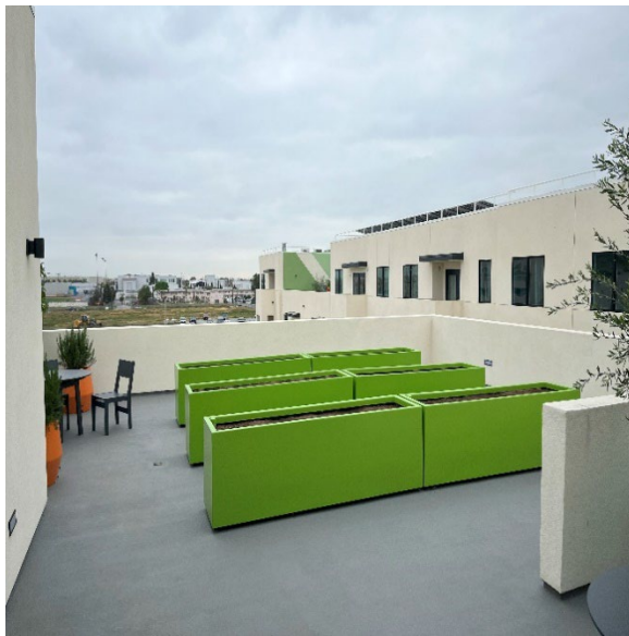
Area S4 - View of building B patio May 7, 2025
