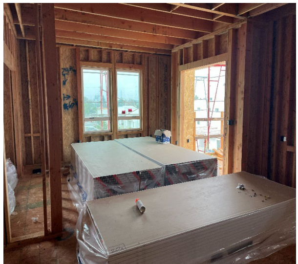
Area S5 - View of Unit November 12, 2025
