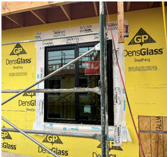
Area S5 - View of Exterior windows November 12, 2025
