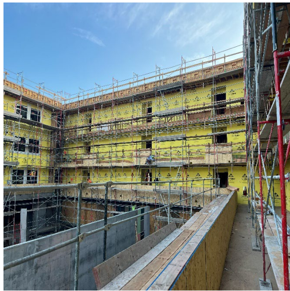
Area S5 - View of exterior west side December 3, 2025
