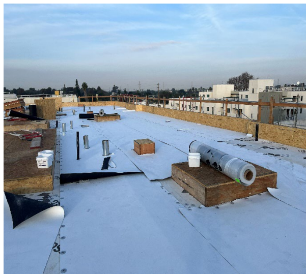
Area S5 - View of roofing install December 3, 2025
