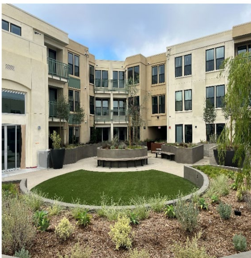
Area H2B - View of Podium building October 2, 2025
