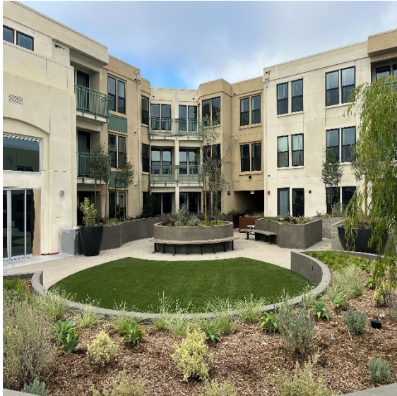
Area H2B - View of Podium building October 2, 2025
