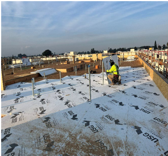
Area S5 - View of roofing install December 3, 2025
