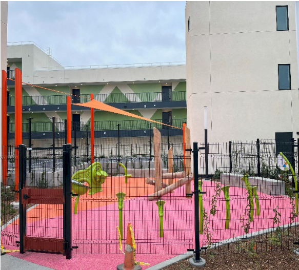
Area S4 - View of building playground May 7, 2025
