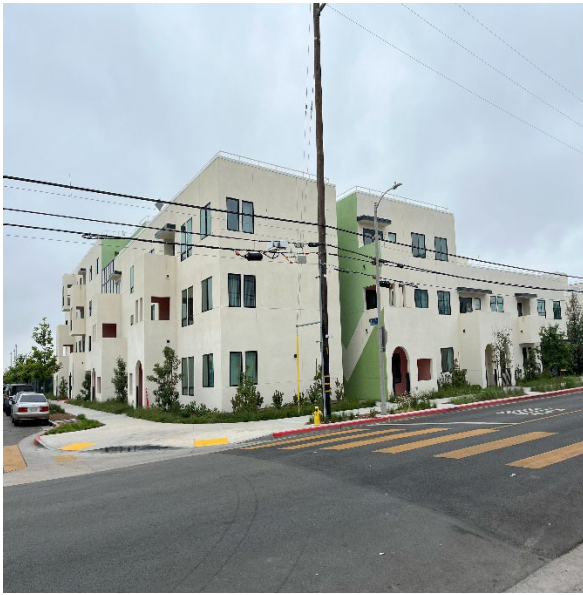
Area S4 - View of building A June 4, 2025
