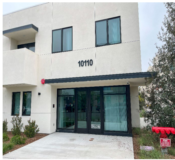
Area S4 - View of building A June 4, 2025
